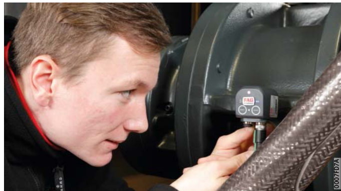
Figure 3 Commissioning of FAG SmartCheck
